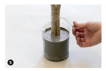
Put the rope into concrete up to the scotch tape marks.
